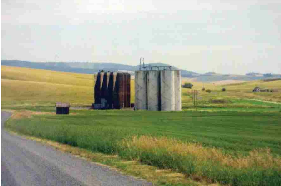
12. Partially dismantled cribbed timber elevator in Garfield, WA
